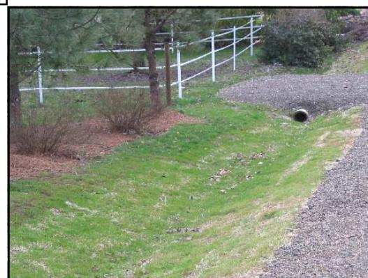
**After:** Graded slope and erosion control fabric permit grass to grow and protect the site from further erosion.
