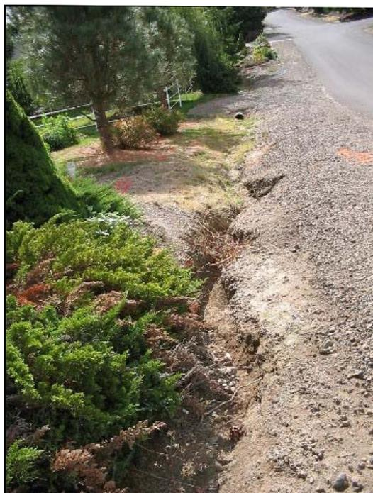
**Before:** Soil erosion along the ditch had occurred after several large storms.
