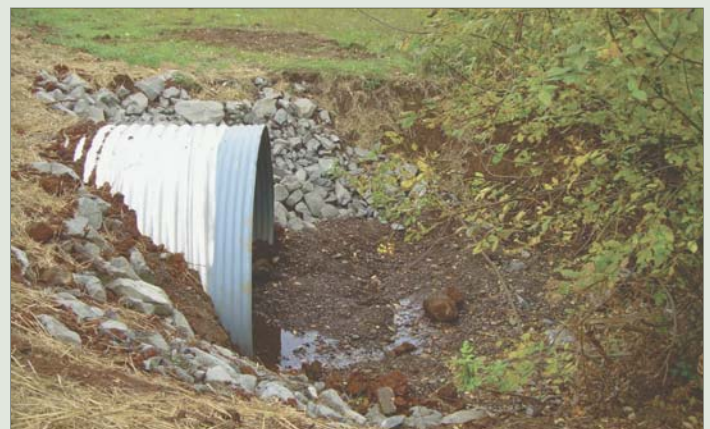
Blair Creek culvert after replacement.
