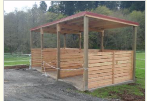
Manure Composting Facility
