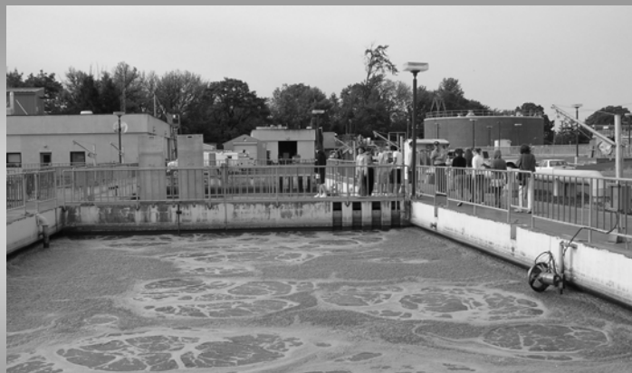
GLORIA SCHOENHOLTZ (CVHS) USED HER MINI-GRANT TO TAKE STUDENTS ON A TOUR OF THE CORVALLIS WASTEWATER RECLAMATION PLANT.
