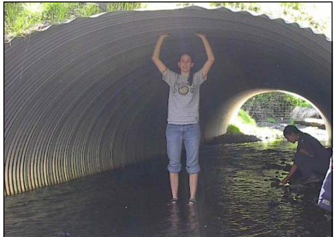
Volunteers assess a Soap Creek culvert in the Luckiamute watershed.
