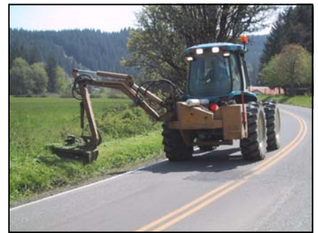
Benton County's Crew clears vegetation from roadside ditches
