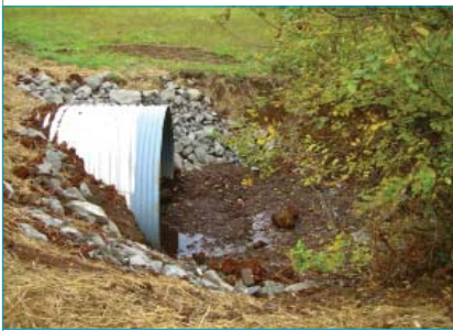
Replaced and countersunk, the culvert now permits fish passage.
