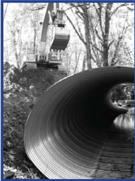
Soap Creek culvert replacement 2005
